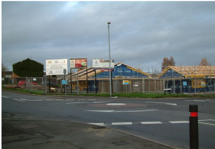
Figure 9: Construction of affordable homes on Austin, Road, Charford
